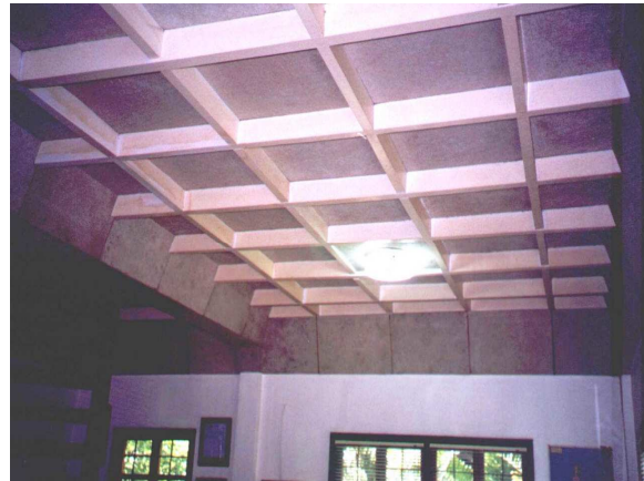
Figure 9 – Interior of house shown in Figure 8 with WSCB-EltoBoard floor, ceiling, and walls (painted)
