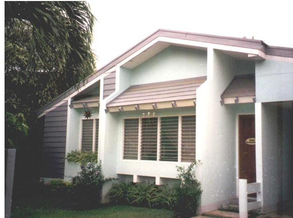
Figure 7 – All exterior and interior walls, floors, and facade cladded with WSCB-EltoBoard (painted)
