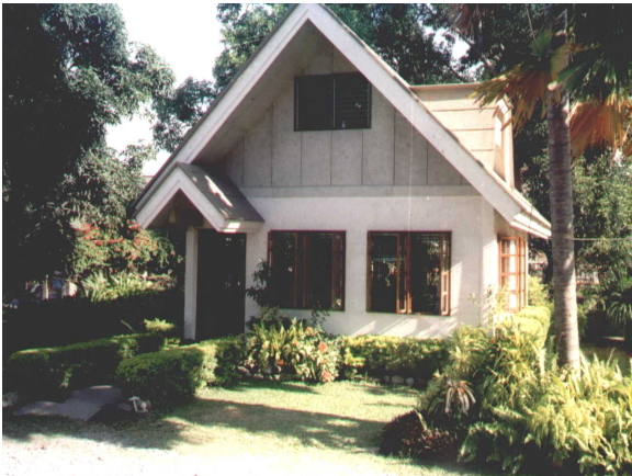
Figure 8 – Two-story house entirely constructed with WSCB-EltoBoard. The exterior ground-floor walls have been stuccoed
