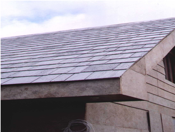
Figure 6 – WSCB-EltoBoard siding and shingles
