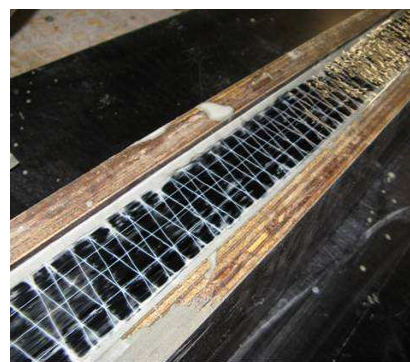
Figure 18 The laid FRP on fresh mortar
