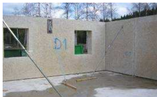
Figure 7 - Installation of Large WWCB Elements
