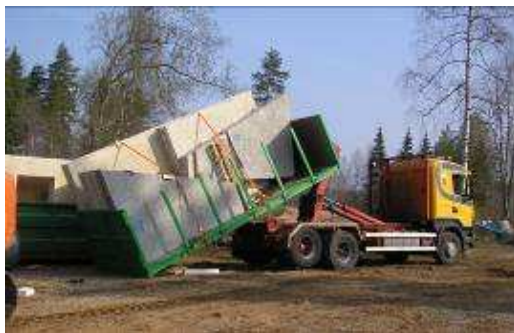
Figure 6 - Arrival of Elements at building site
