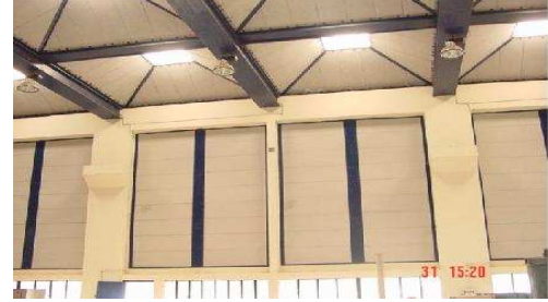
WALLS & ROOF - Figure 3
