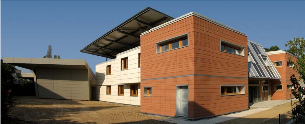
The experimental building in Northern Italy, seen from the South-West corner.
