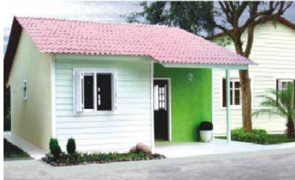
**Figure 17 – Example of application of non-asbestos fiber-cement flat sheets and corrugated roofs.**
