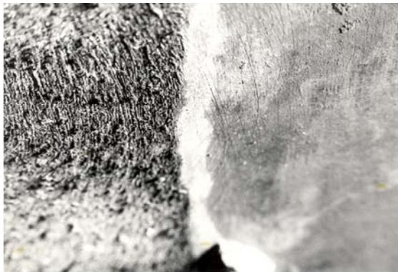
A single old asbestos cement roofing tile. On the left the area of tile exposed to the elements and on the right the area of tile covered by the overlapping tiles.
