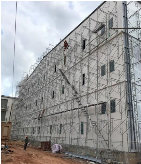
Figure 2: Building walls using sandwich panels
