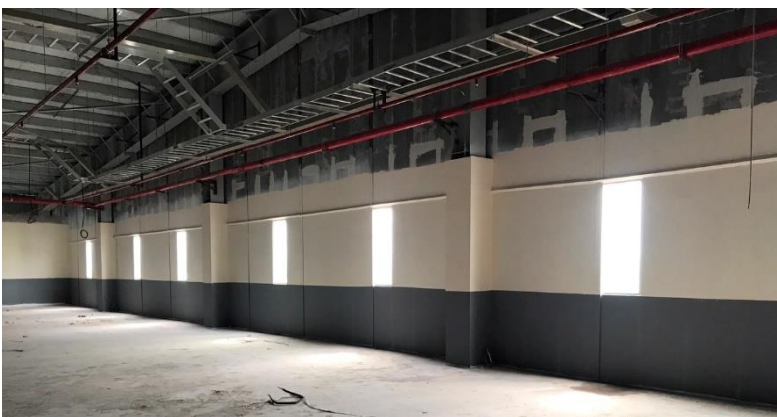
Figure 3: Partition walls using sandwich panels
