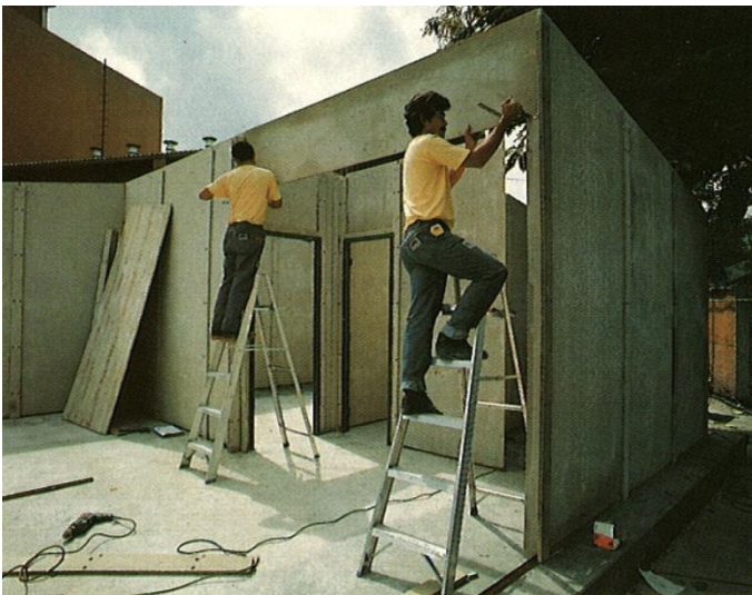
The metal door and window frames are installed.
