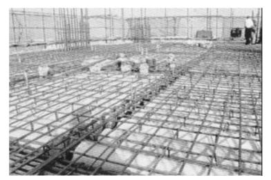
Figure 9- GRC tube-shaped formworks used in cast-in -place reinforced concrete cavity floor
