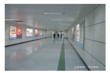
Figure 2—'Kafu' boards used as interior walls in the South Station of Shanghai Subway line
