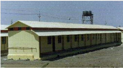
DISASTER SHELTERS - Figure 2
