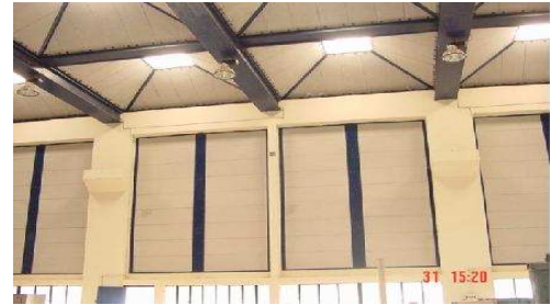
WALLS & ROOF - Figure 3
