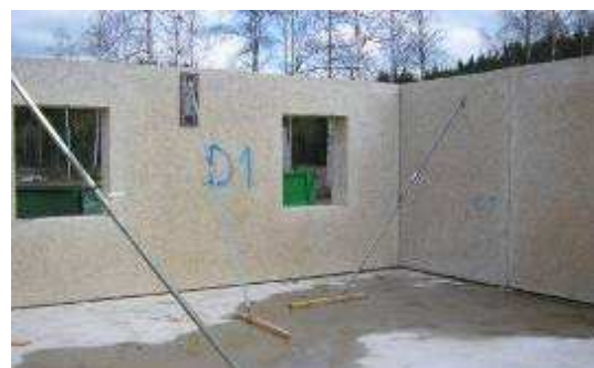
Figure 7 - Installation of Large WWCB Elements
