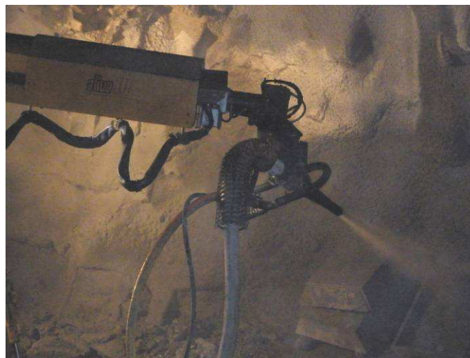
Figure 4 – Testing under field conditions: shotcrete application with bi-component fibers.
