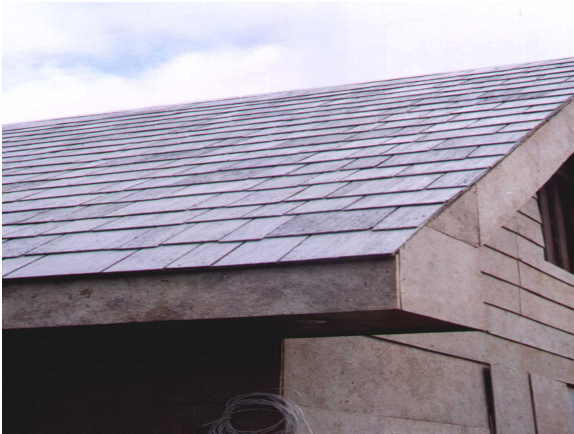
Figure 6 – WSCB-EltoBoard siding and shingles
