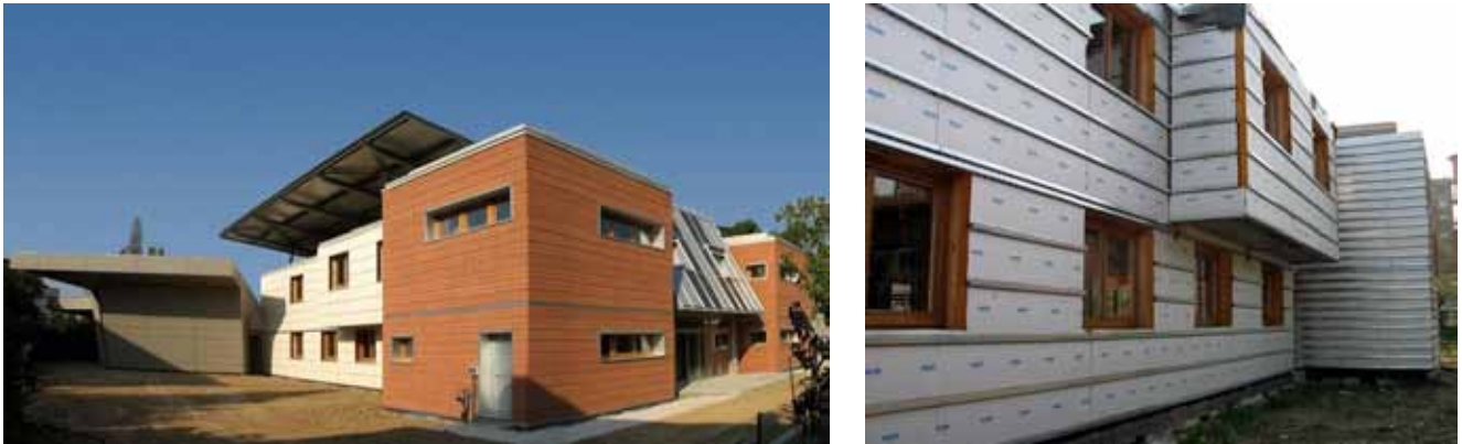
Figure 7 – The finished building from the south-west (left) and the multi-functional insulation panel before the installation of the fibre-cement cladding (right).
