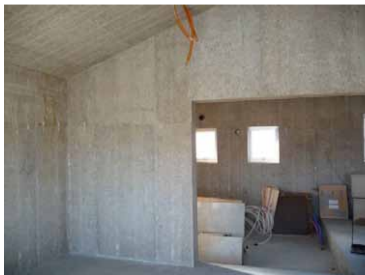
Figure 10 - EltoBoard applied in walls, floors and roof
