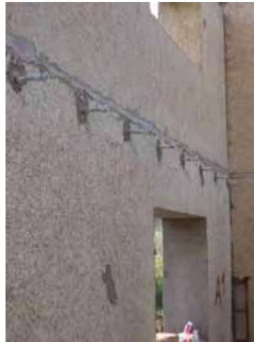
Figure 17 - Anchors in ring beam for floor
