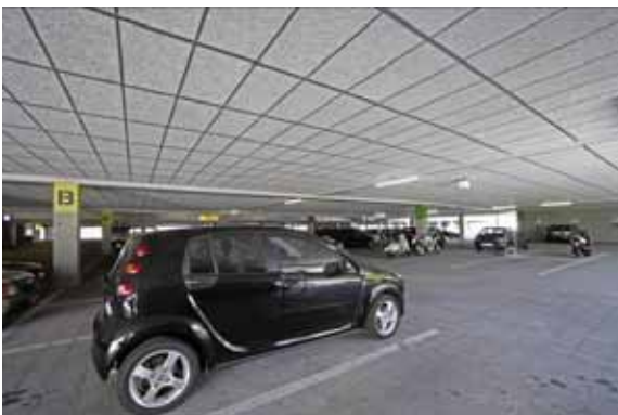
Figure 5 - Acoustic ceiling panels (WWCB)
