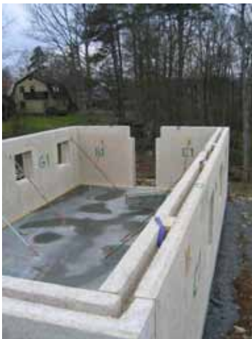
Figure 16 - Open Ring- beam
