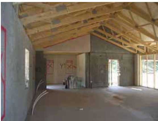
Figure 19 – Inner walls prior to stuccoing
