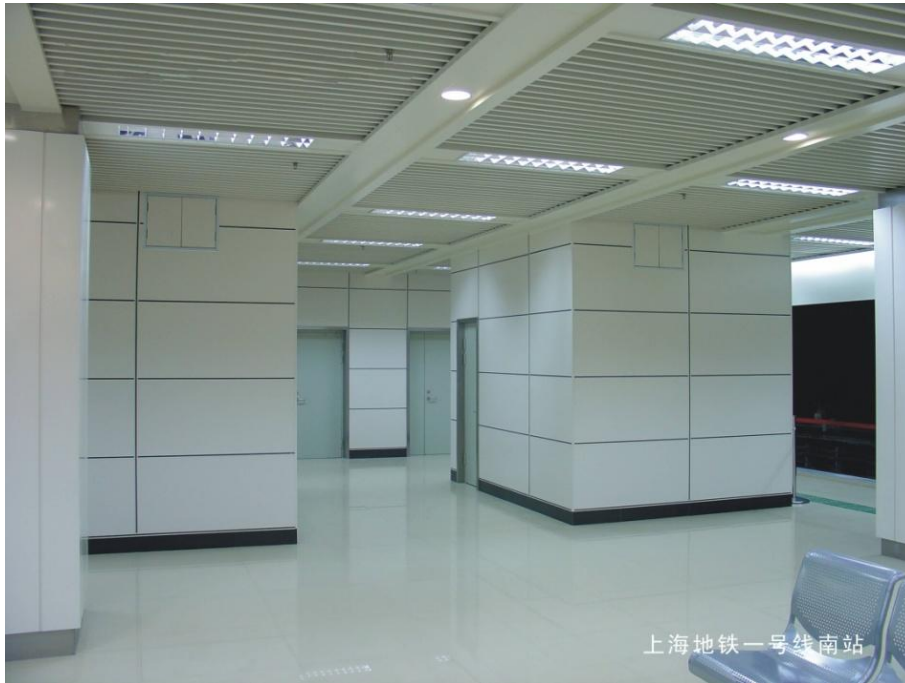
Figure 5: Internal application of fibre cement sheet
