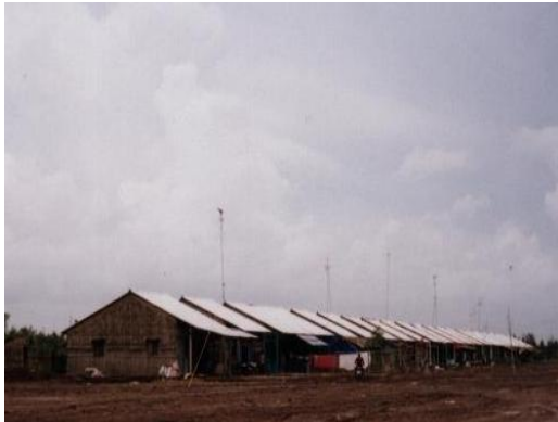
Figure 11: PVA roof sheets in Vinh Chau , Soc Trang Province
