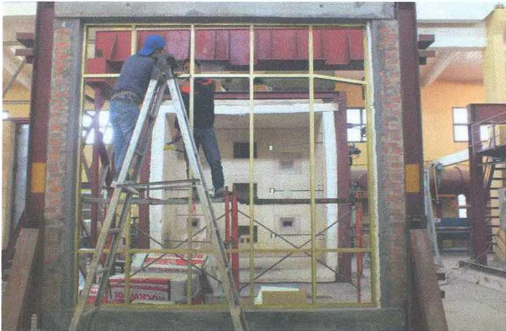
Figure 7: Installation of the steel stud system of the specimen
