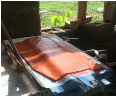
Figure 4: Moulding of Roofing Tiles
