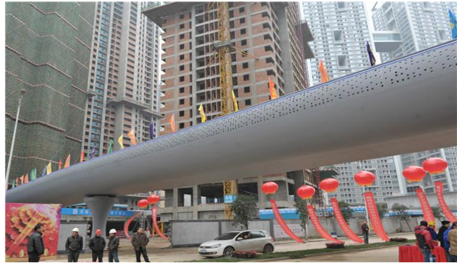
Fig. 9 Assembly precast UHPC bridge in Changsha
