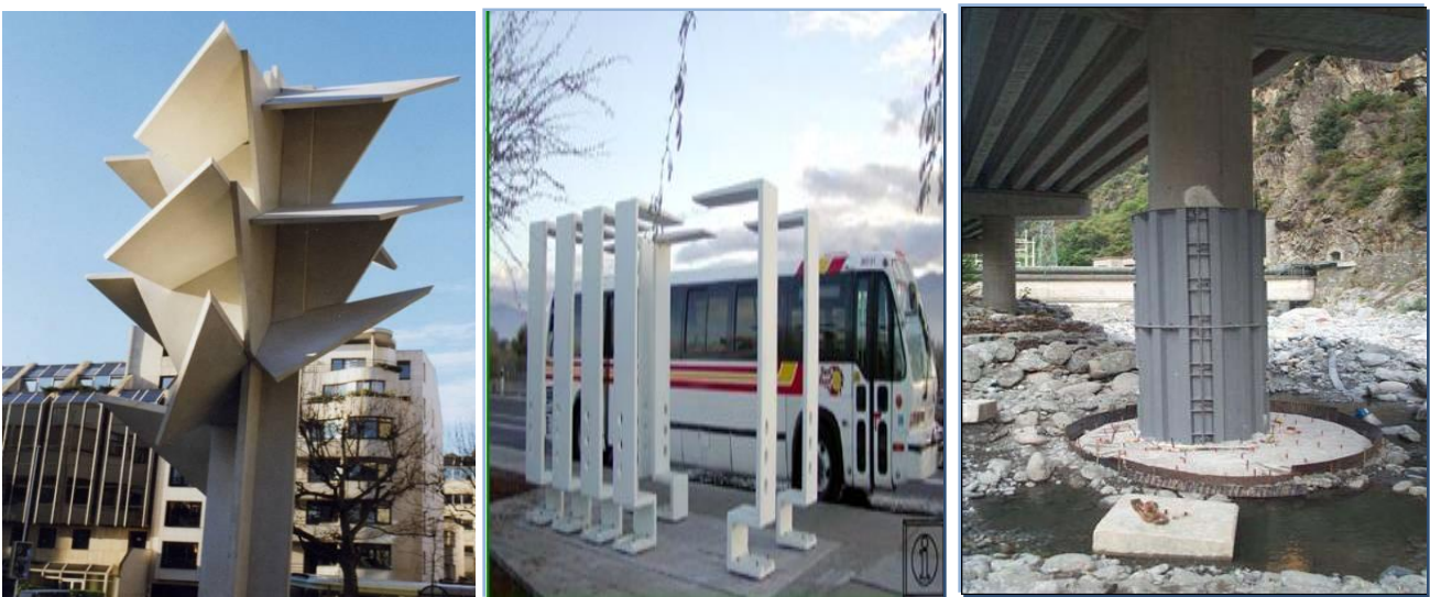
(a) Precast structure
