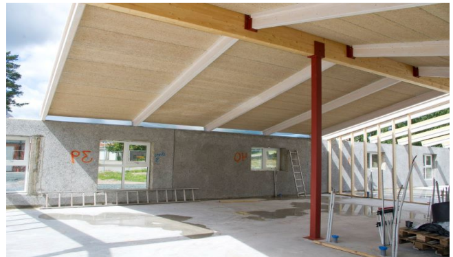
Figures 51, 52, 53, 54 – Construction of a highly insulated day-care centre in Sweden, utilising Large Elements for the outer walls and Reinforced Roofing Boards for the roof (Träullit, Sweden)
