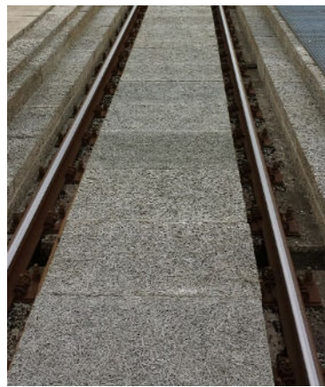
Figure 24, 25 – WWCB Elements placed between the tracks of a light-rail overpass
