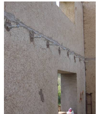
Figure 44 - Anchors in ring beam for floor support
