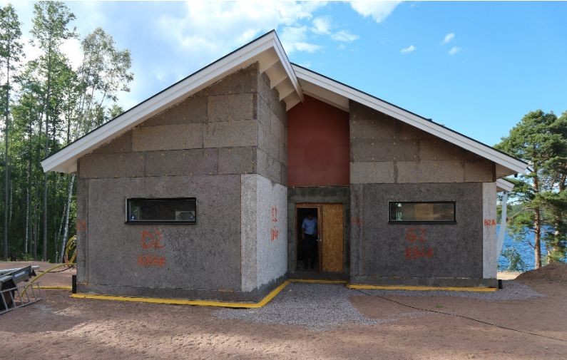
Figures 45, 46, 47, 48 - two-story villa under construction (Träullit, Sweden) ....
