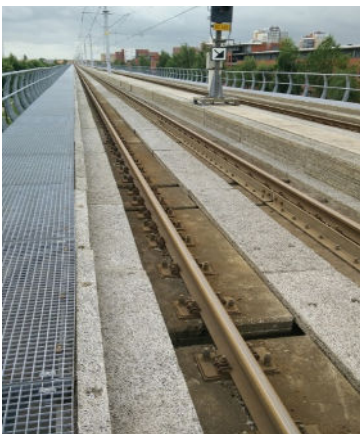
Figure 24, 25 – WWCB Elements placed between the tracks of a light-rail overpass
