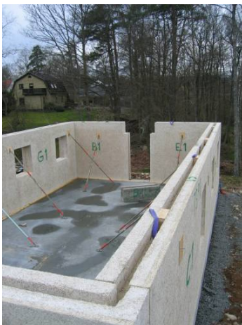
Figure 42 - Open Ring-beam
