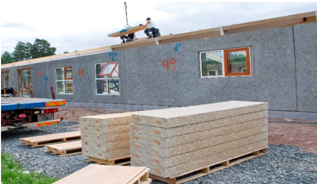
Figures 51, 52, 53, 54 – Construction of a highly insulated day-care centre in Sweden, utilising Large Elements for the outer walls and Reinforced Roofing Boards for the roof (Träullit, Sweden)
