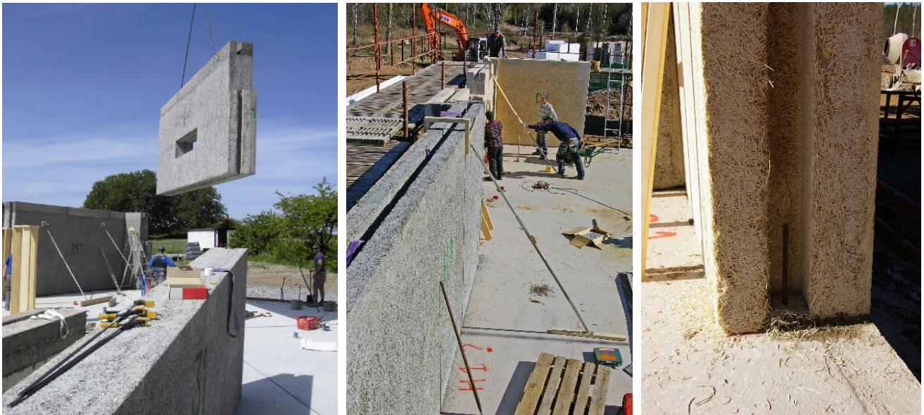
Figures 39, 40, 41 - Ready Elements are efficiently placed on the ready concrete slab (Träullit, Sweden)
