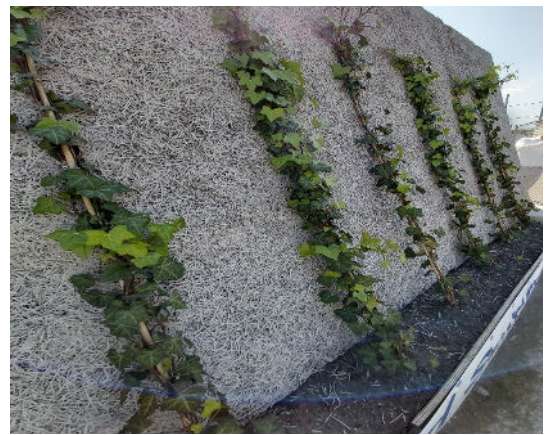
Figure 26 – WWCB Sound Barrier being covered by ivy for a natural look
