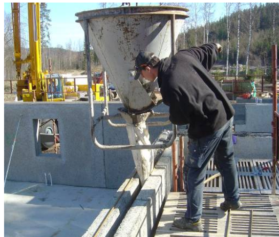
Figure 43 - Pouring of concrete
