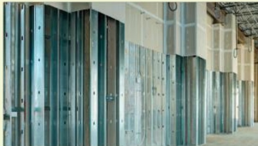
Column & Beam Encasements
